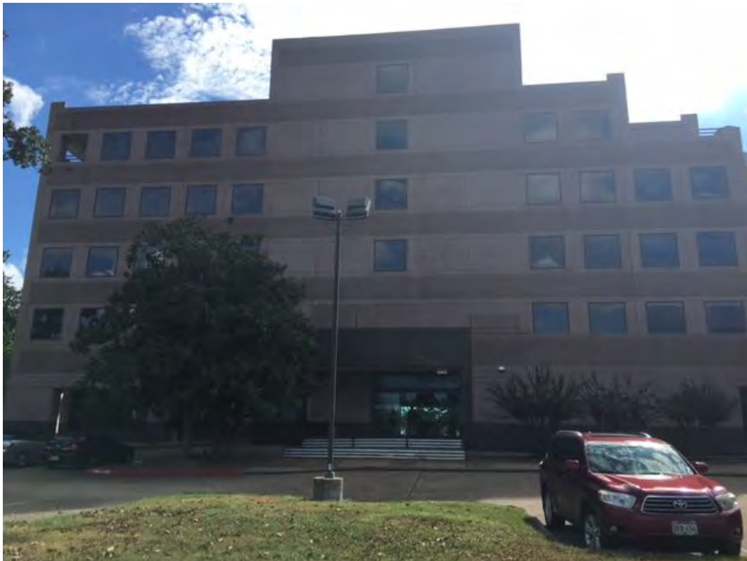
Looking East at Subject Property
