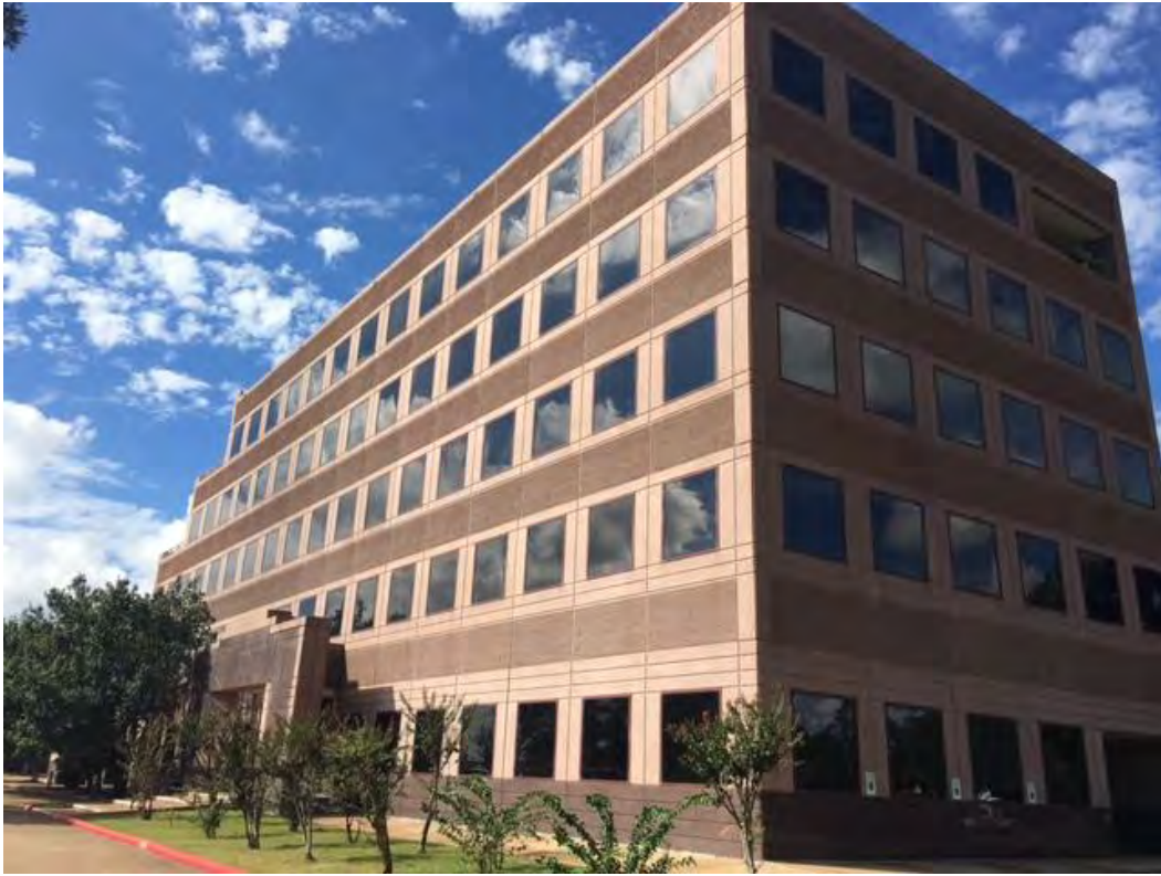
Looking Southwest at Subject Property
