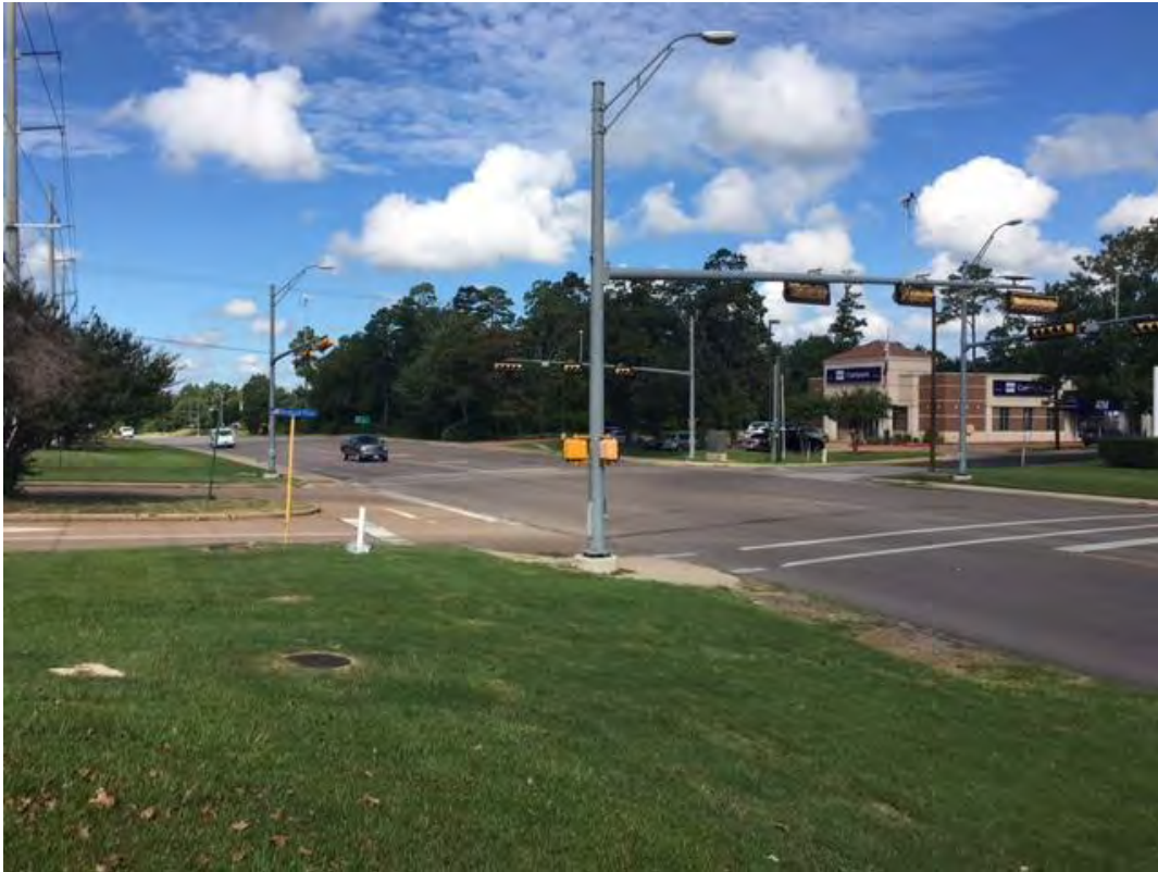
Looking West along State Highway 30
