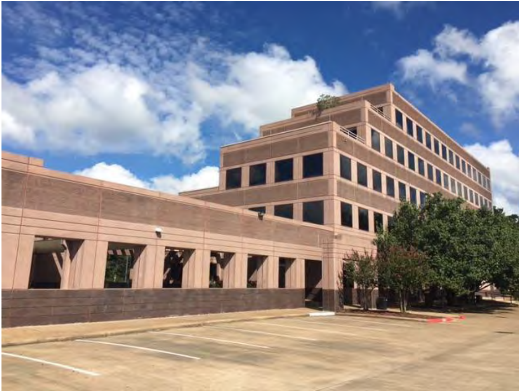
Looking Northwest at Subject Property
